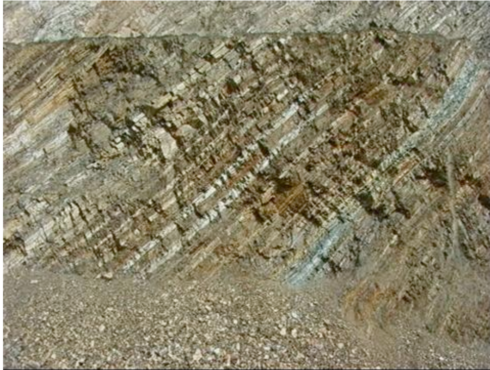
Figure 3. Weak waste material
